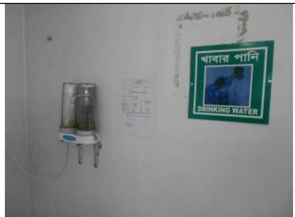
Drinking water point
