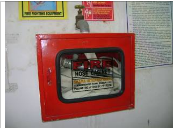
Fire hose pipe
