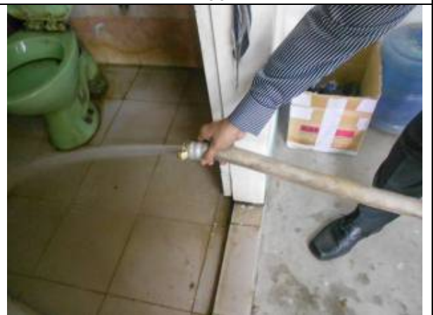
Sufficient water pressure in fire hose pipe
