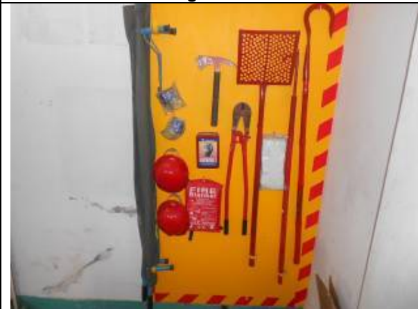
Fire fighting equipments
