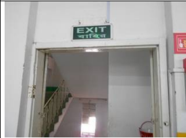
Exit sign is marked
