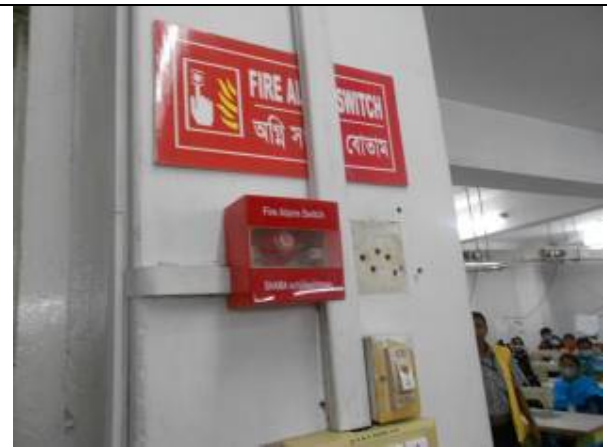
Fire alarm switch
