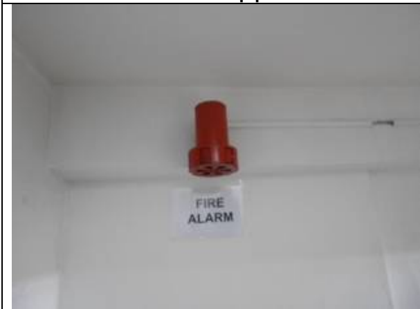
Fire alarm bell
