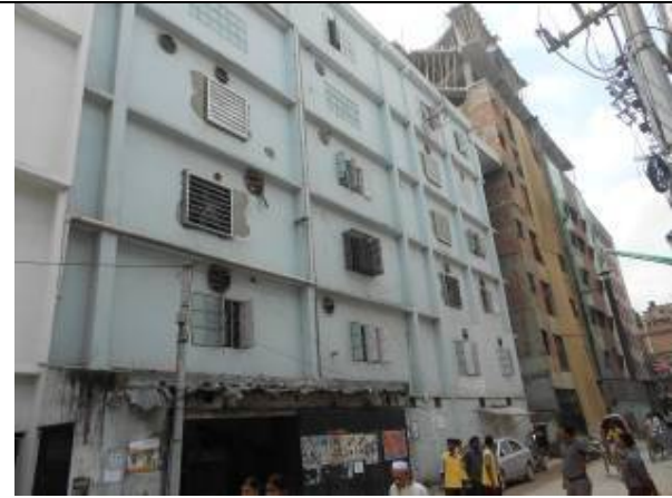
Front view of factory building
