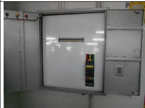
Inner insulator was provided inside the electric control panel
